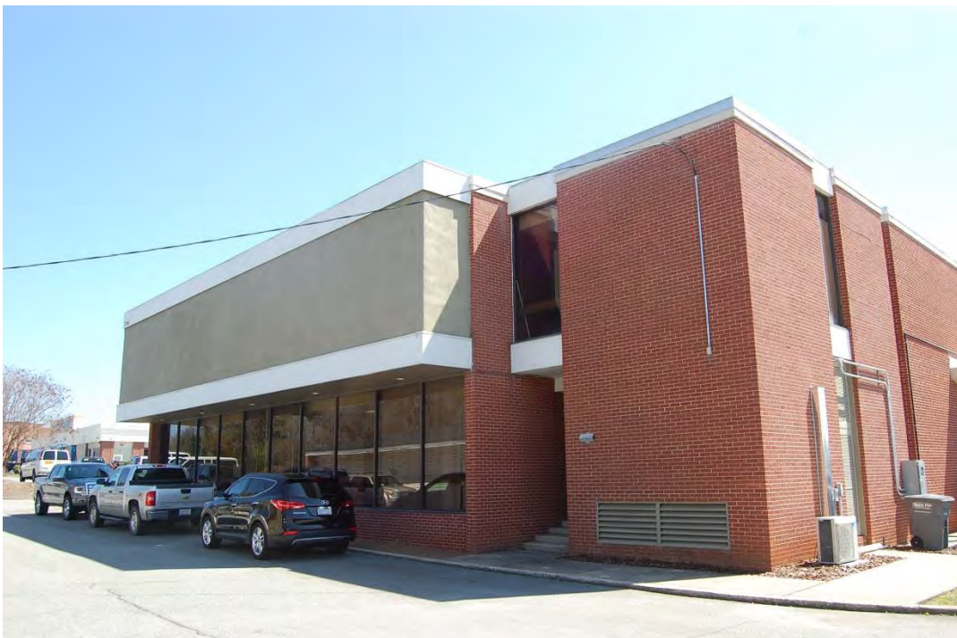
Landsdale Corporation Building, ca. 1970 Rear Addition Showing Stuccoed Second-Floor Windows, Looking Southeast.
