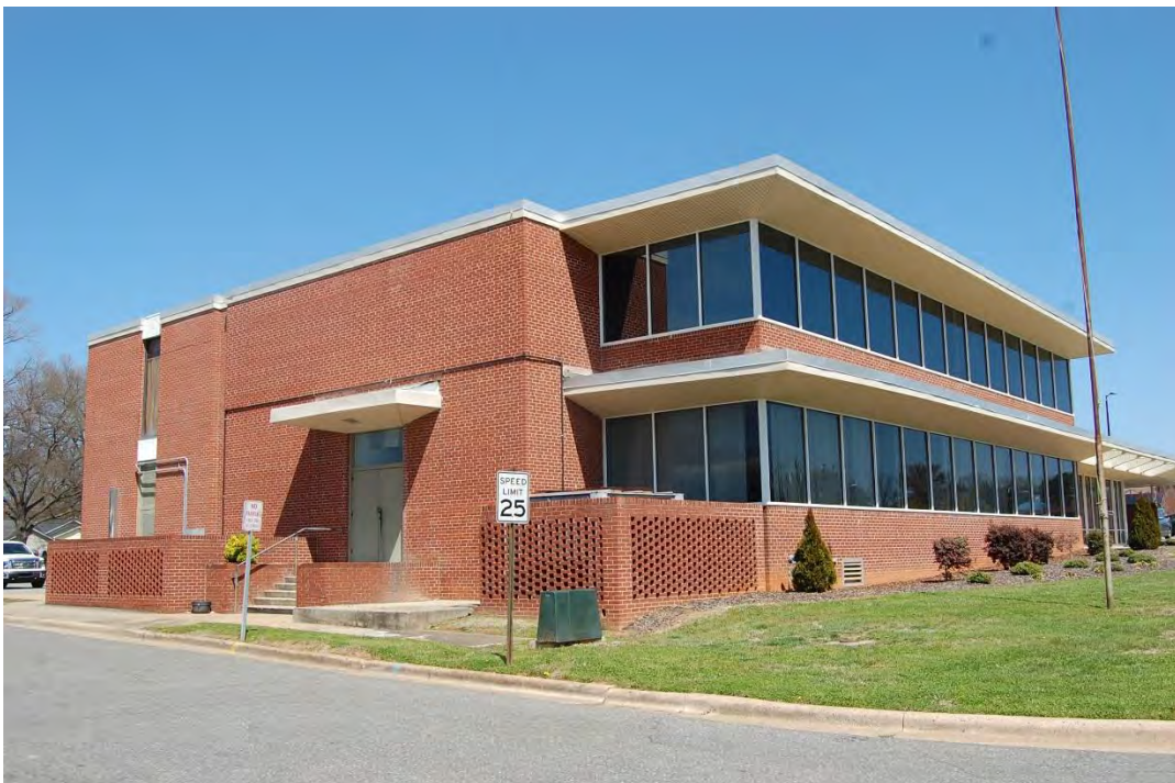
Landsdale Corporation Building, Façade and Side (West) Elevation, Looking Northeast.
