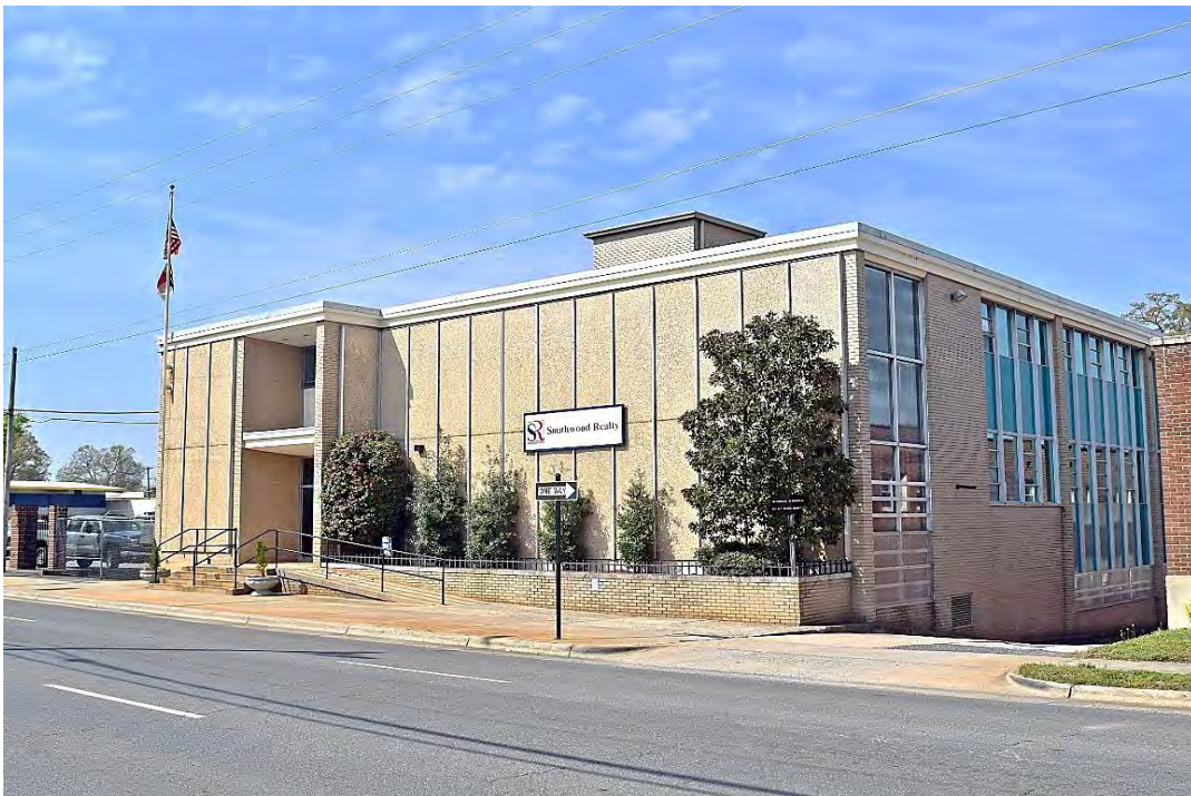
Gaston County Department of Public Welfare Building, 1957, 165 South York Street, Gastonia.
