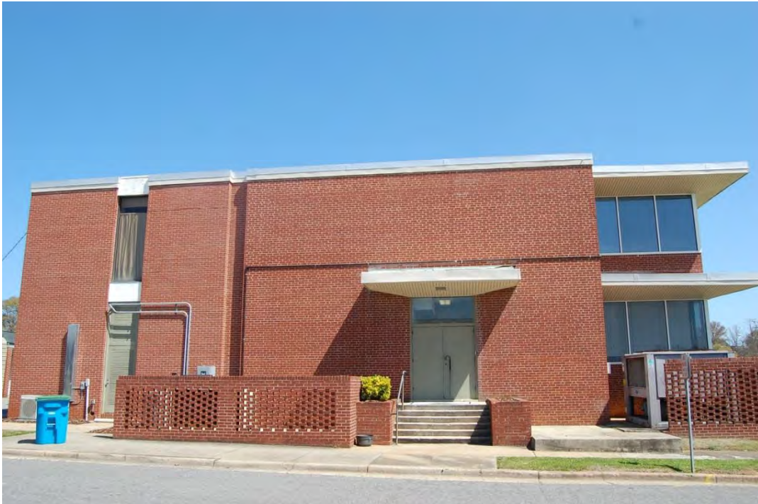
Landsdale Corporation Building, ca. 1954 Building (Right) and ca. 1970 Rear Addition (Left), Side (West) Elevation, Looking East.
