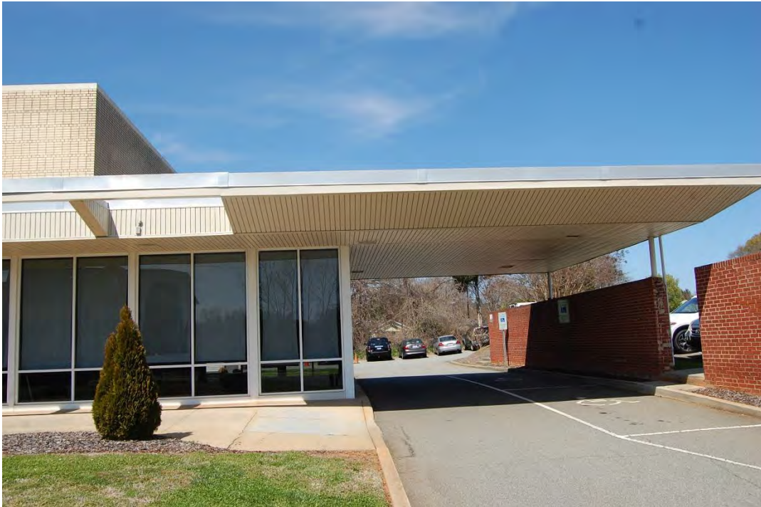
Landsdale Corporation Building, One-Story Wing and Drive-Through Canopy, Looking North.
