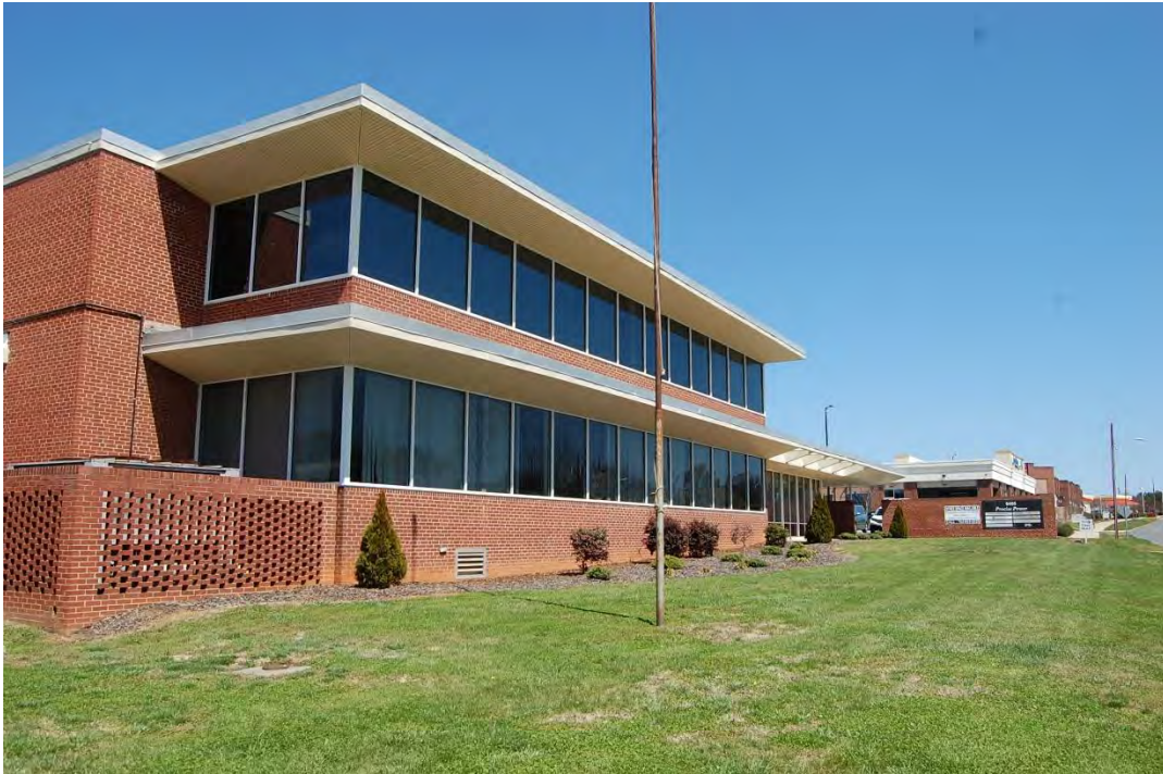
Landsdale Corporation Building, Façade, Looking East.
