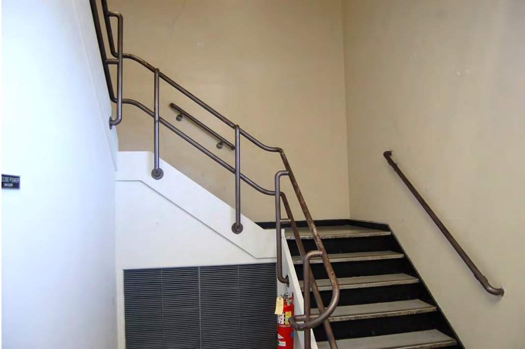
Landsdale Corporation Building, Interior, Staircase.
