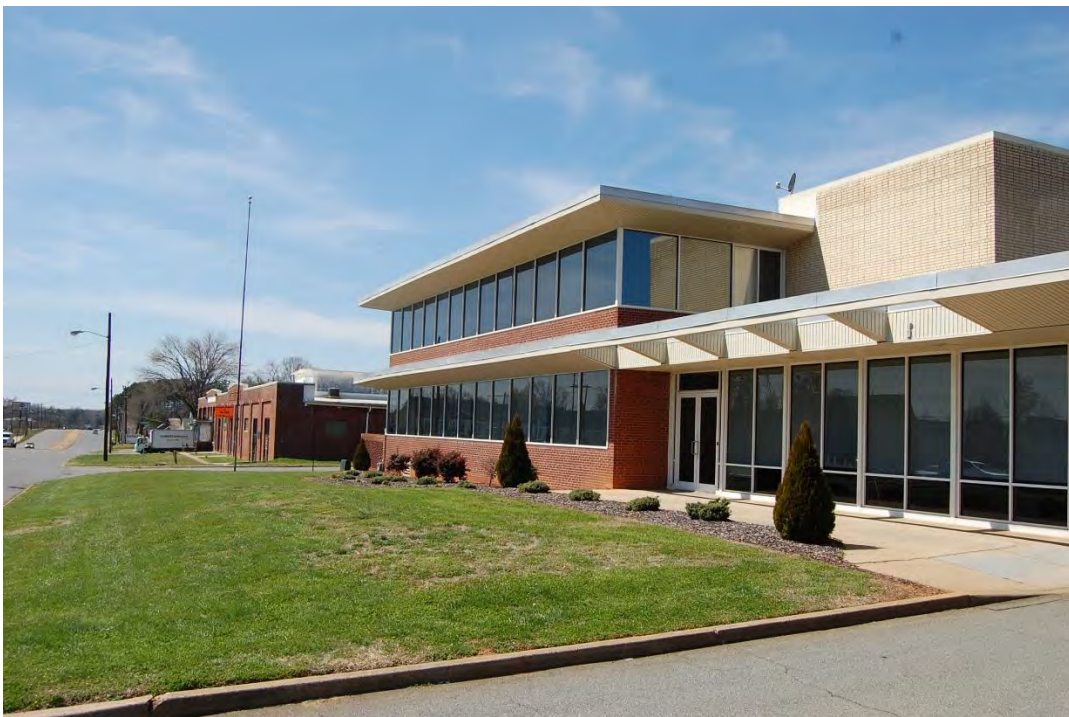
Landsdale Corporation Building, Façade, Looking West.
