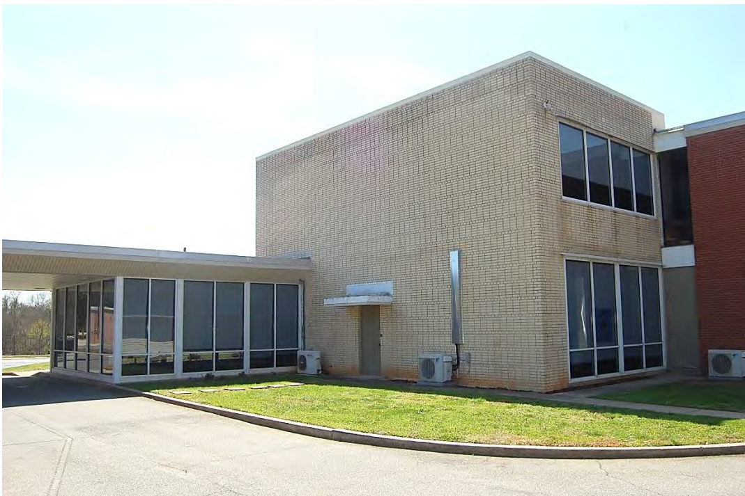
Landsdale Corporation Building, Side (East) and Rear (North) Elevations, Looking Southwest.
